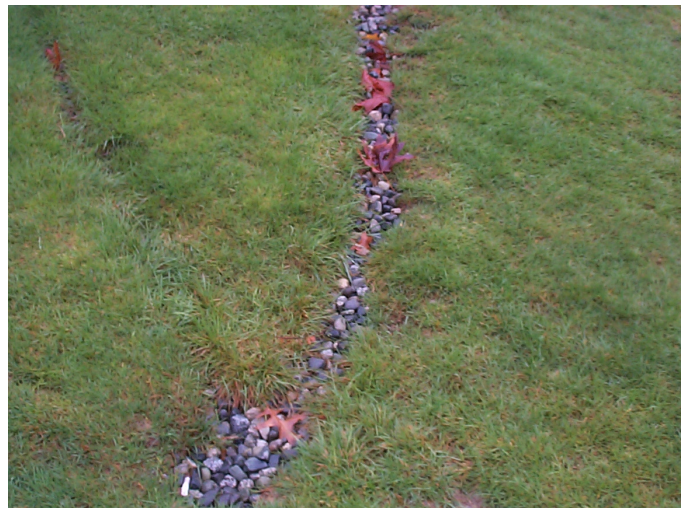
Surface curtain drain
